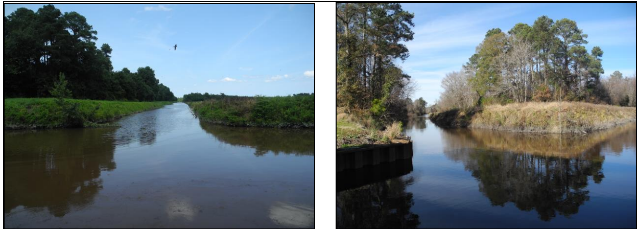
FIGURE 4-12. Photograph of the intersection of two primary canals designed to lower the water table by about 5 feet for agricultural development.
