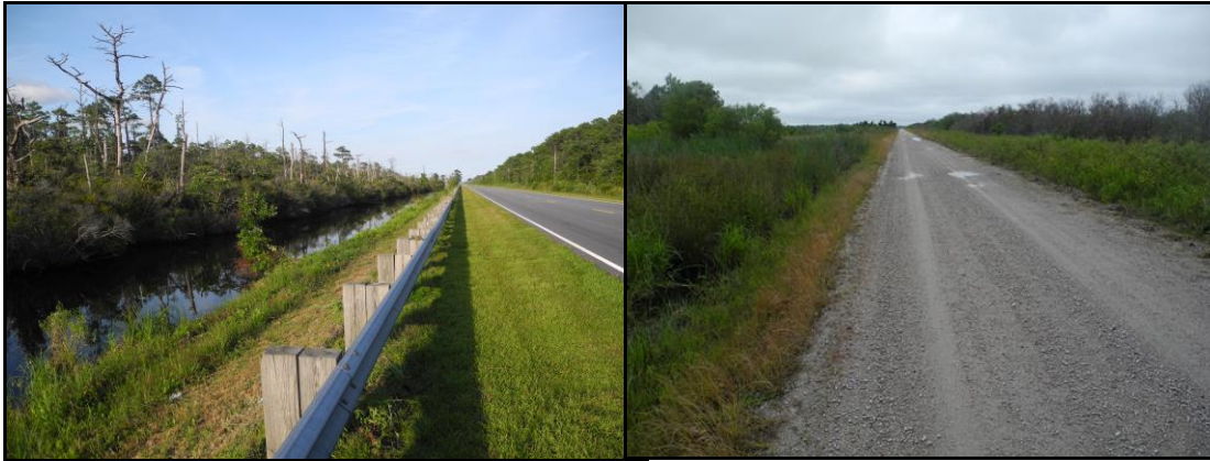
FIGURE 3-17. The main canals and collector ditches excavated within the Albemarle-Pamlico Peninsula have either a highway, farm road, or field path adjacent to it that was built from the removed sediment.
