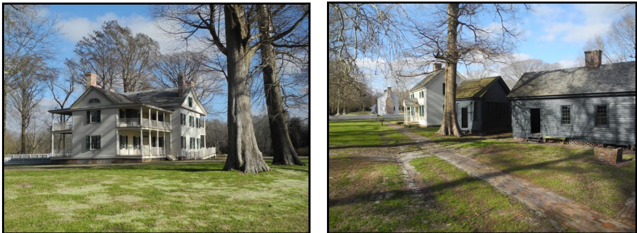
FIGURE 4-10. Photograph on the left shows the restored plantation house that was the home of Josiah Collins III at Somerset Place Ca. 1837. The right-hand panel shows (from left to right) the restored hospital, school house (which is the visitor’s center today), laundry, and cook house.
